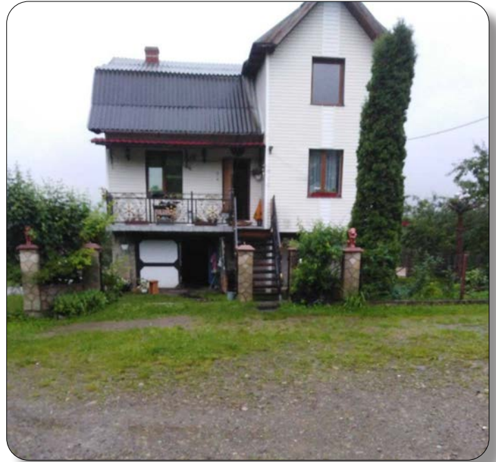
Picture of house before flood.
